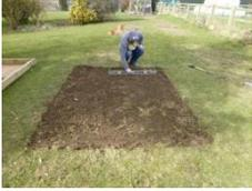
Clear and prepare a firm, level area slightly larger than the size of your ProBase. ProBase can be laid directly onto a sub-base of grass, gravel or bare soil. For guidance on how to prepare a suitable sub-base please call our helpline.
