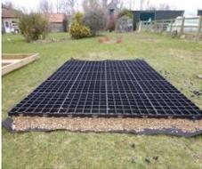
Lay out your grids, making sure the feet are facing down. Interlock the grids and secure using the fixing pegs which you can detach from the side of each grid. Four per grid. The grids can be cut to size using a hand saw.
