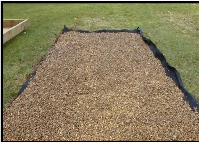
Sub Base made from Pea Gravel
