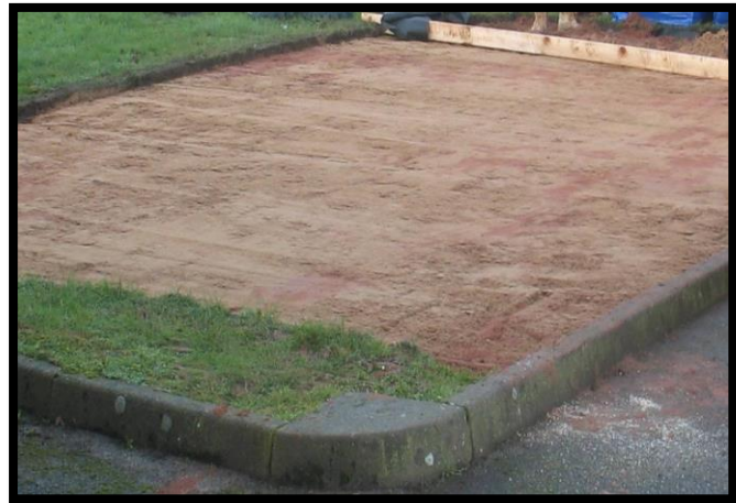
For heavy buildings, fill with 10mm round Pea Gravel
