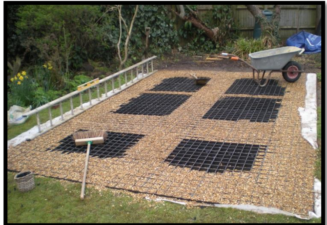
For heavy buildings, fill with 10mm round Pea Gravel
